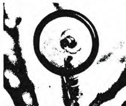
The break can be seen in the center of the vacuum tool just before the pressure is applied to force the chemical into the air space.
